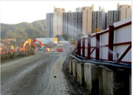
Mist sprayers are installed along haul road.
