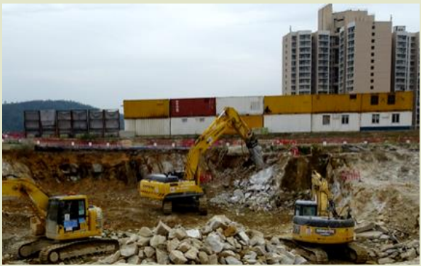
In addition to erecting noise barriers, containers between rock breaking area and nearby residential area can further reduce construction noise effectively.
