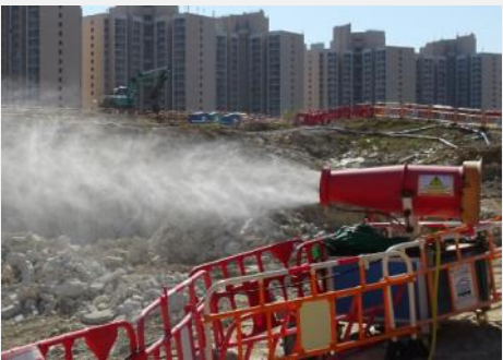
Mist cannons are placed in the construction site.
