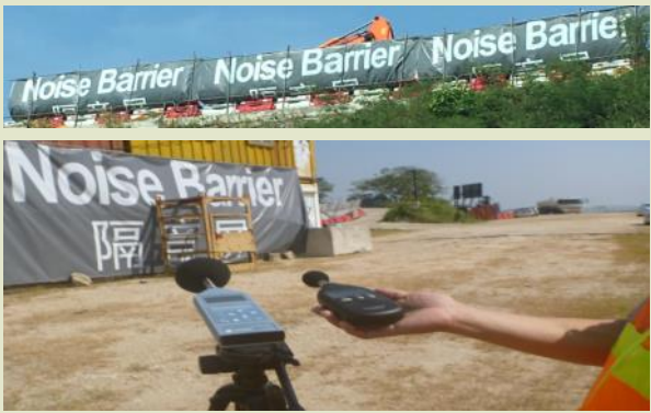
Noise barriers are erected on site to mitigate noise nuisance to residents.
