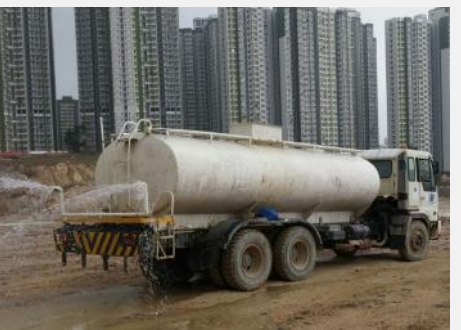
Spraying regularly by water trucks in the construction site.
